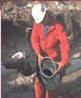
Figure 3. Steel spacer ring for flange connection.
