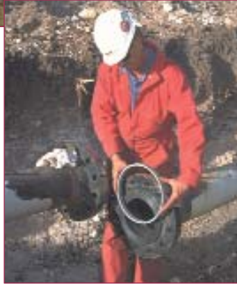
Figure 3. Steel spacer ring for flange connection.
