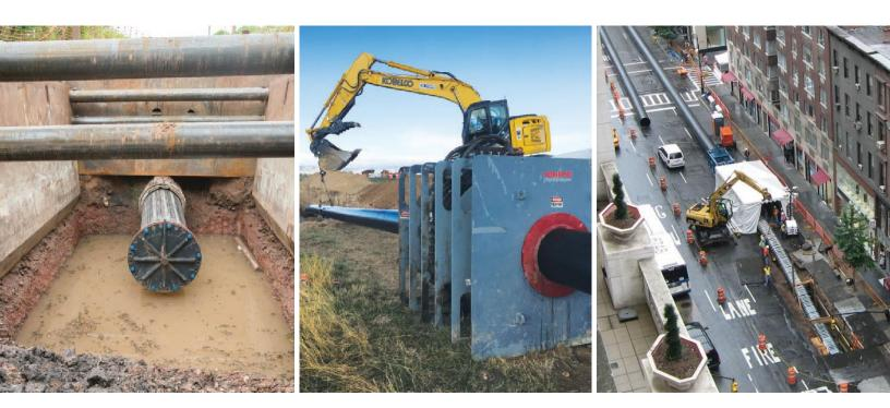
Much of the world's pressure pipe infrastructure is long past its design life or is in need of repair. Complete replacement of these pipes using conventional dig and replace solutions can be time consuming, costly (up to 3 times the cost of insitu rehabilitation) and very disruptive to traffic, the general public and the environment. These problems can easily be avoided by choosing the Tite Liner® system—a close-fit, high-density polyethylene (HDPE) solution for pipe renewal.
