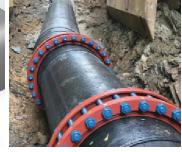
The Tite Liner® system is suitable to connect to all types of piping systems (DIP, CS, PCCP, AC, HDD, etc). Fittings, valves and miters can be accommodated with HDPE, DI, CI or other materials and bolt directly to the Tite Liner® system.
